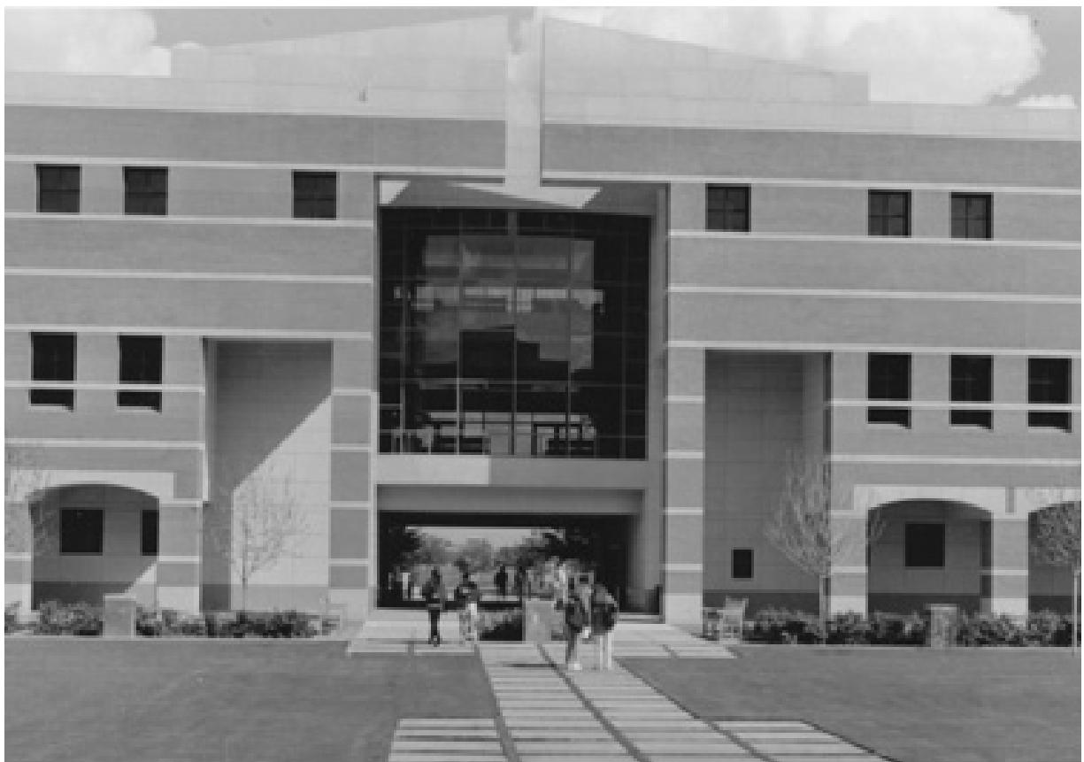
ASU West Classroom Laboratory/Computer Building
