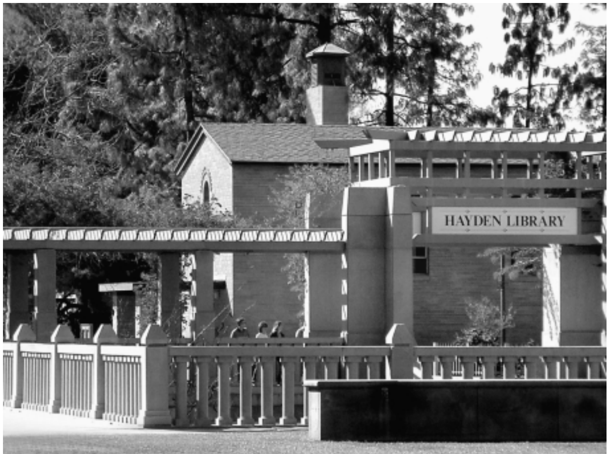
Stairwell to the underground entrance of Hayden Library
