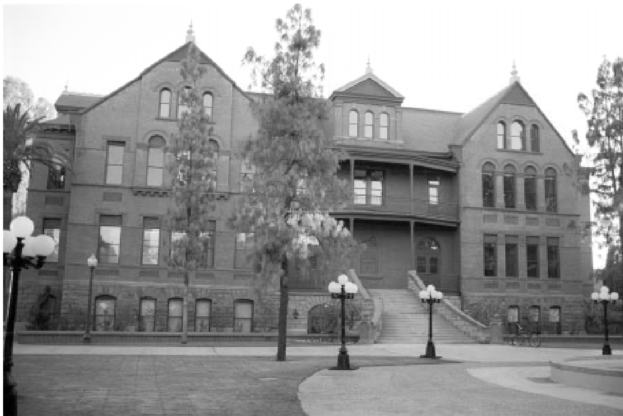
Old Main after the completed restoration of 2000
