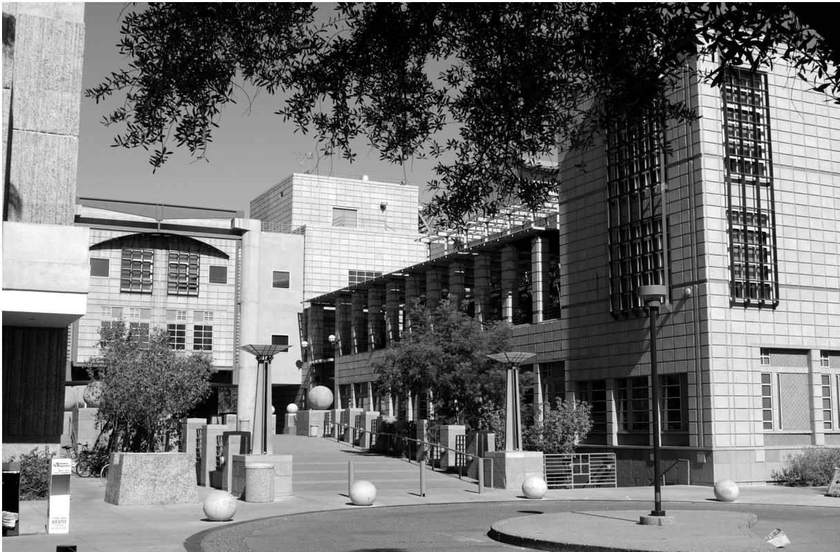
The College of Architecture and Environmental Design/North building
