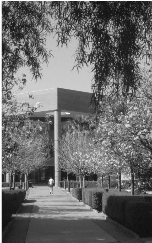
The Student Services Building
