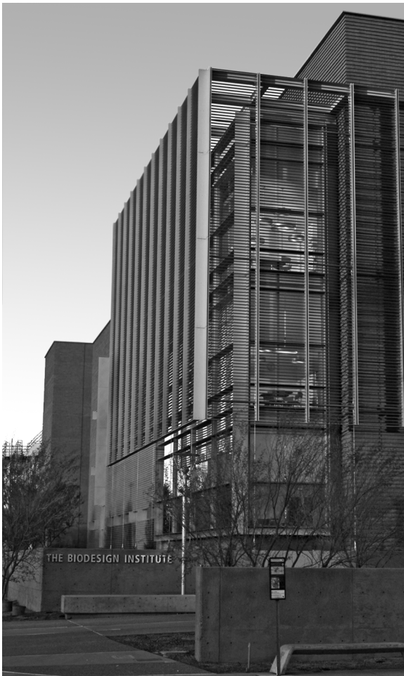
Biodesign Institute Building A was recently completed. The complex will include three additional buildings. Tim Trumble photo
