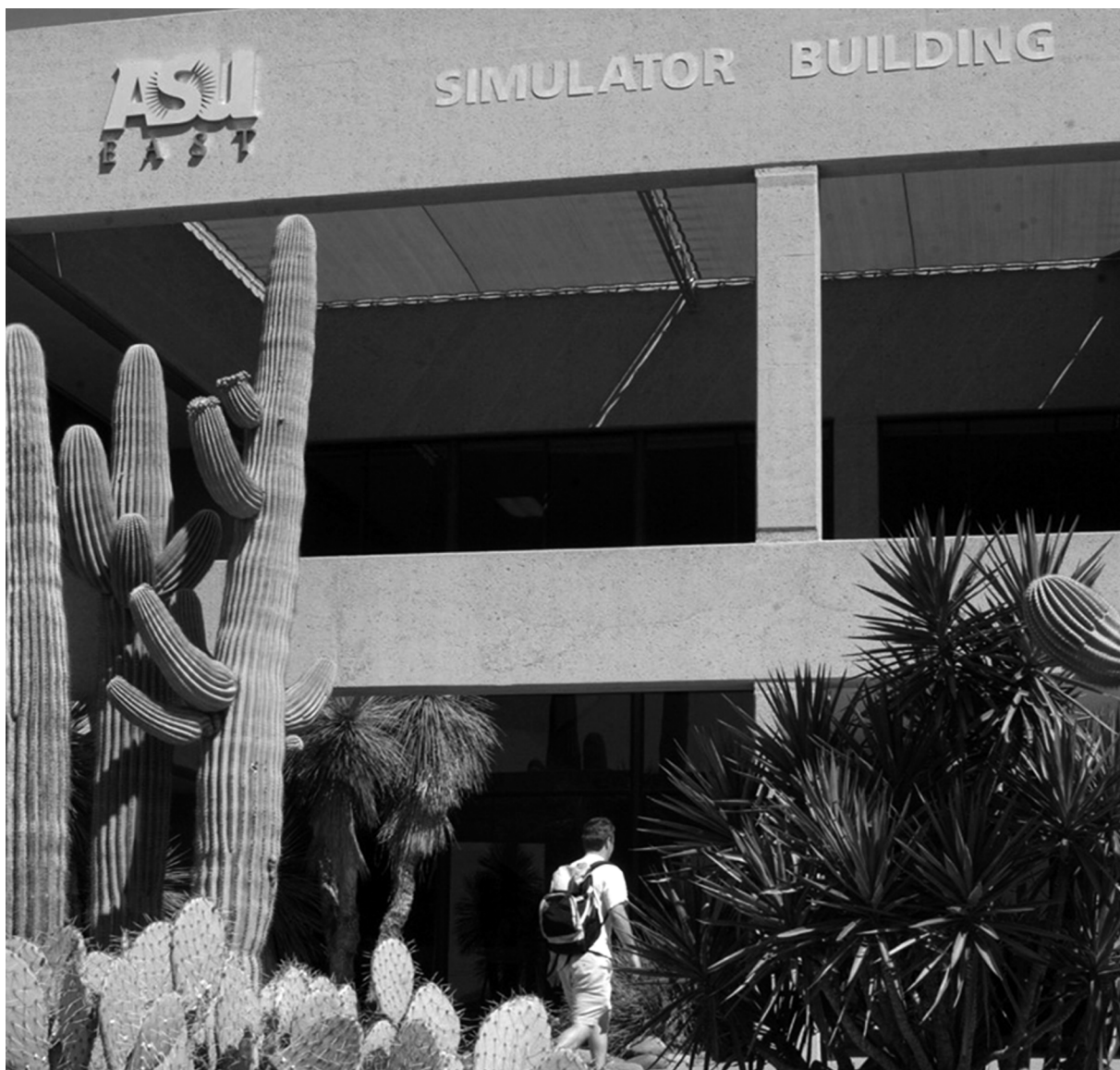
The Flight Simulator Building is a prominent facility for East campus Master of Technology programs.
