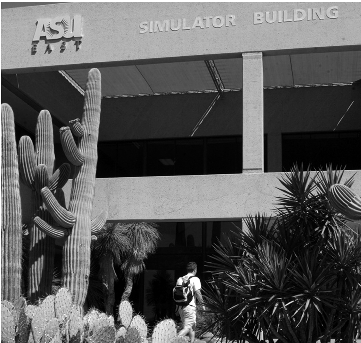
The Flight Simulator Building is a prominent facility for East campus Master of Technology programs.
