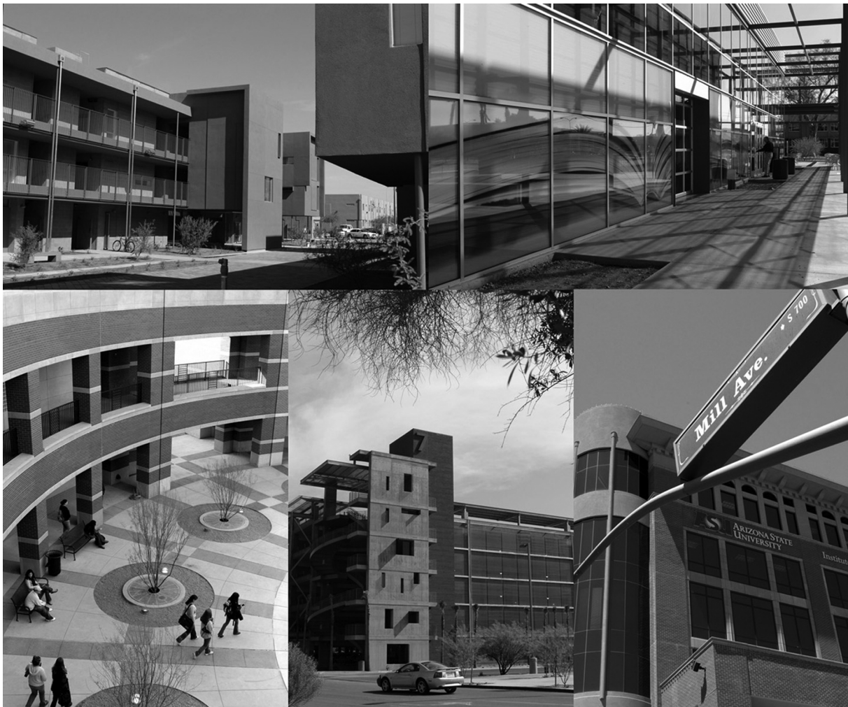
New buildings continue to emerge on ASU campuses. Facilities that opened in 2004 include, clockwise from top left , Adelphi Commons II on the Tempe campus, Williams Campus Union on the East campus, the Brickyard on Mill at the Tempe campus, Parking Structure 7 on the Tempe campus, and CLCC II on the West campus.
