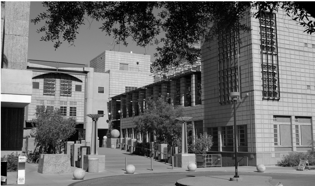
The College of Architecture and Environmental Design/North building
