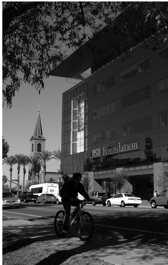
The ASU Foundation building, which opened in January 2005, is home to the university's administrative offices.
