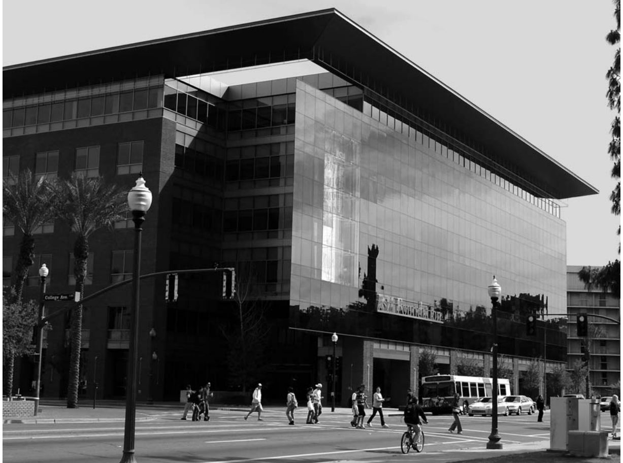
ASU Foundation Building
