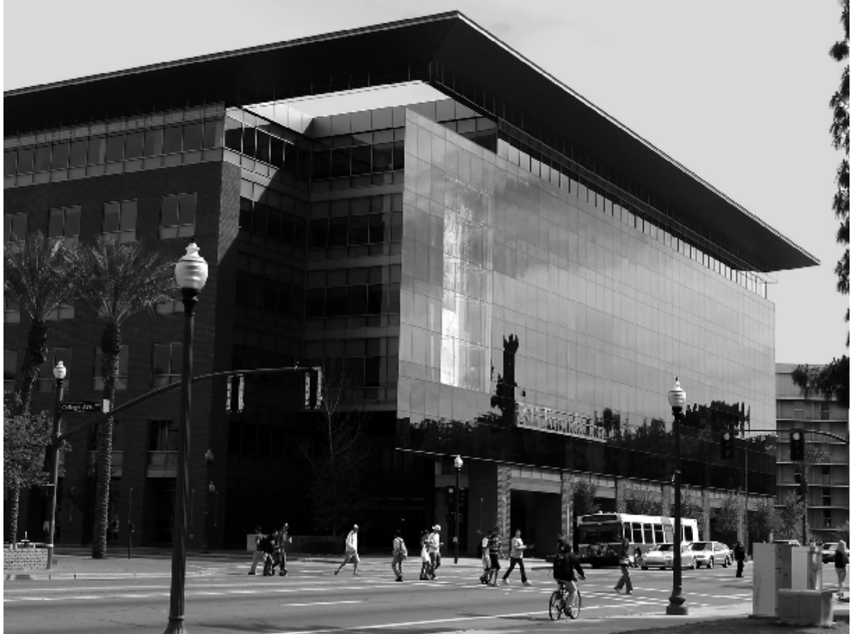
ASU Foundation Building
